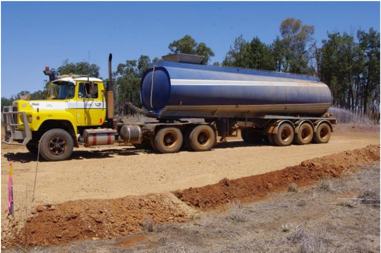
Figure 4: Wetting down of first layer of road base. Indicates surveyor's pegging.
