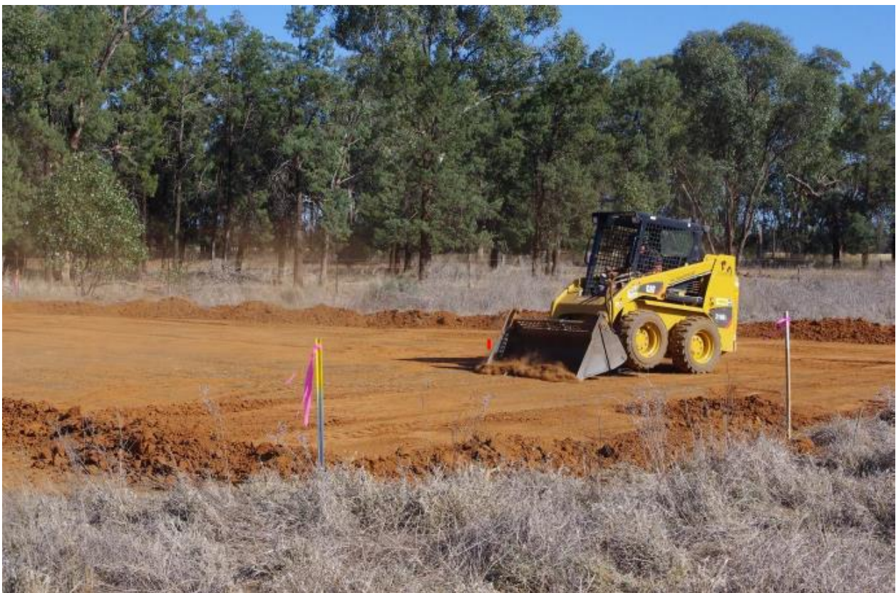
Figure 3: Photo showing bobcat stripping topsoil, looking west.
